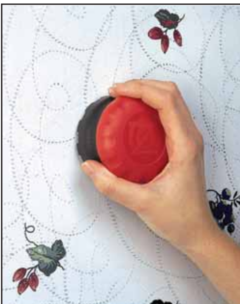
Scoring will allow wallpaper stripper to loosen the glue behind the wallpaper and make it easier to remove.
